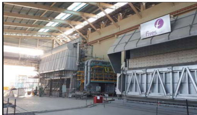
Figure 2. The twin chamber furnace (left) and one of the two tilting, melting/holding furnaces (right) being installed at the recycling plant (June 2017).
